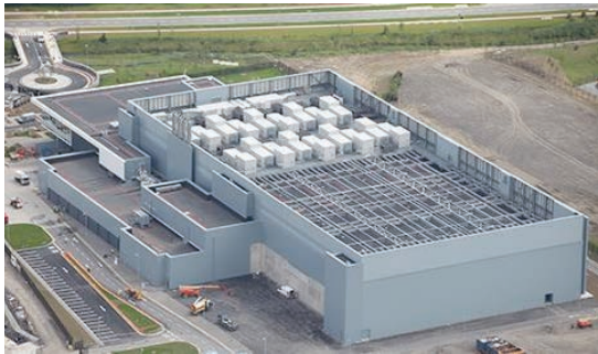
Example of a Microsoft Datacenter in Ireland
